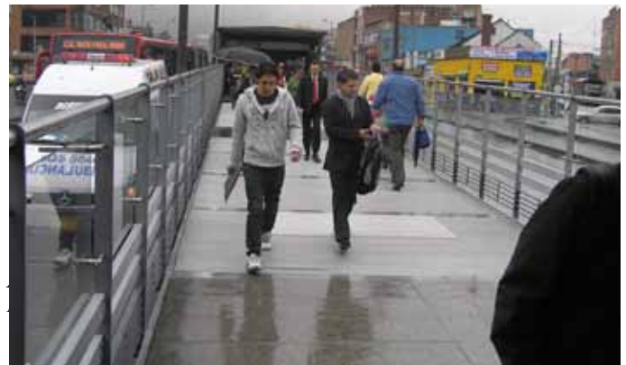
TransMilenio 2011: the guardrails along the pathways were raised to make it more difficult to climb over. We recommend using this higher type of guardrail on any pathway connecting different parts of the same station. EMBARQ photo.
